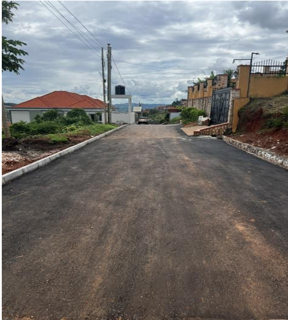
Newly tarmacked section of Podocarpus Street done privately by residents.
