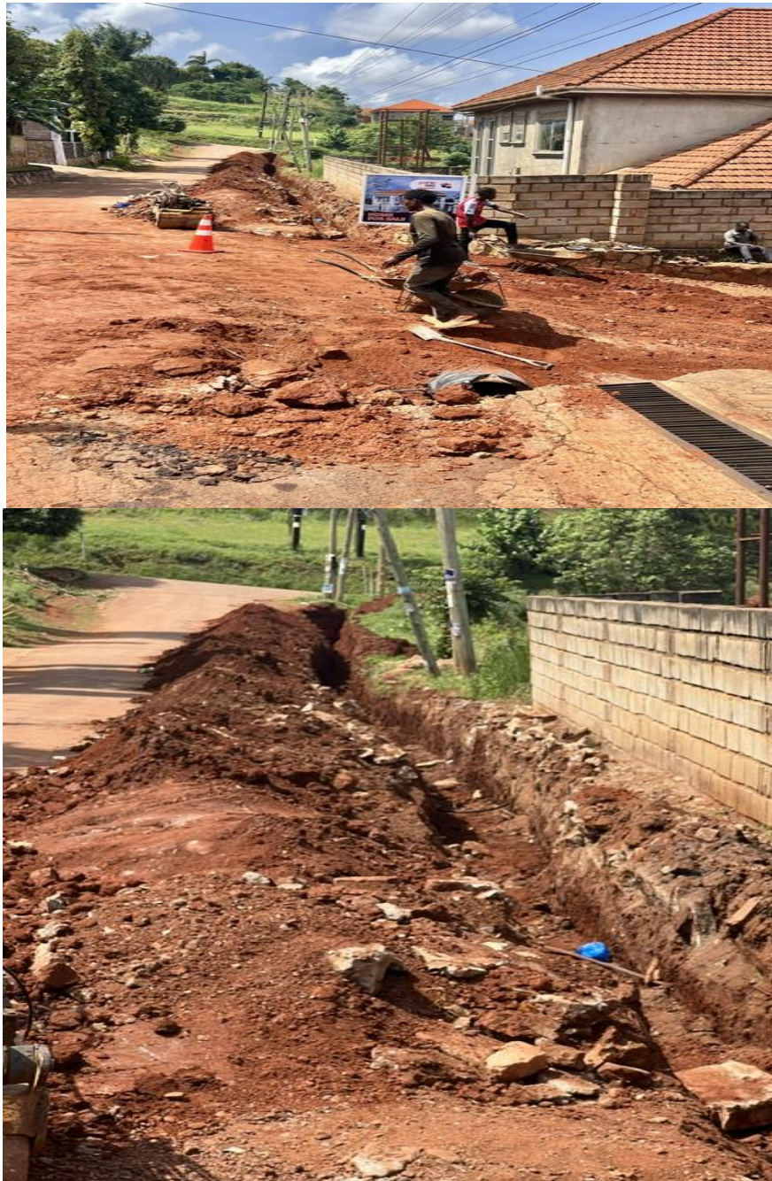
Ongoing Drainage works on Pear Lane
