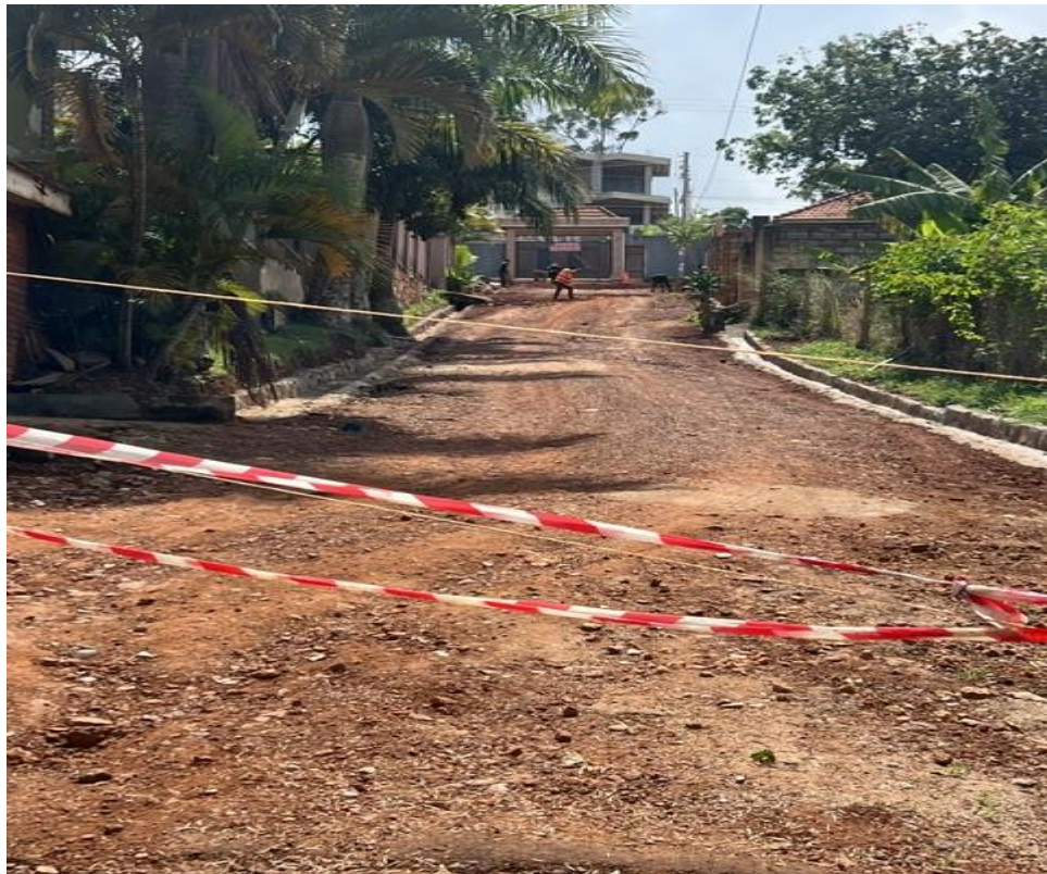
Apple/Podocarpus road works underway and 80% complete
